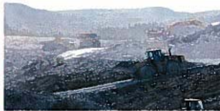
Plant Site Leveling
