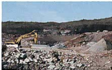
Storm Water Channel Development
