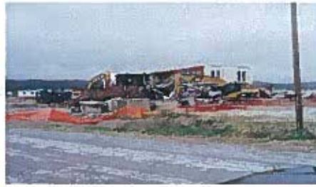
Demolition of Administration Building
