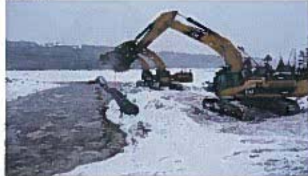
Intake pipe installation for Camp Water Supply
