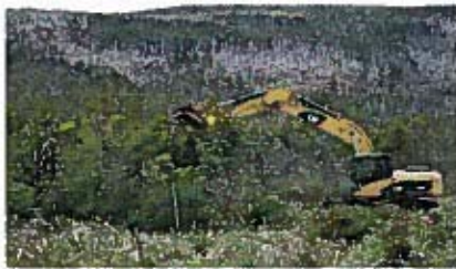
Clearing Access Road
